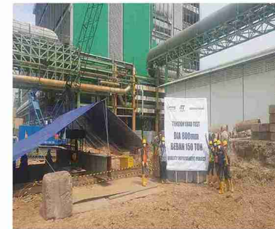
Tension Loading Test "Reaction System"
